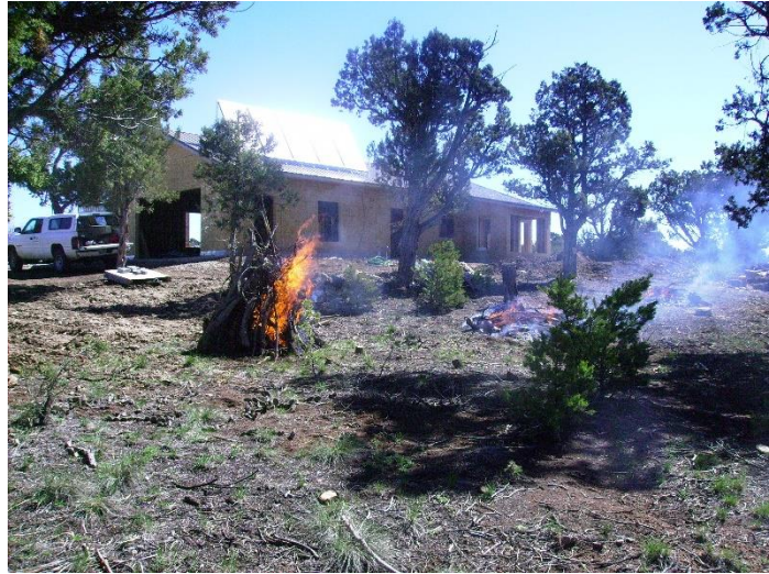
Fuels Mitigation and Defensible Space Creation during Home Construction
